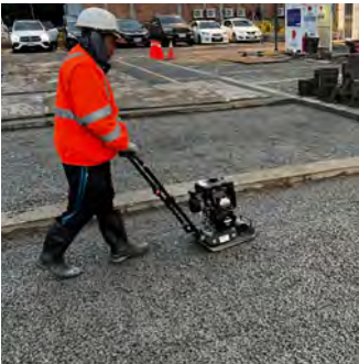
Strengthening Construction with the "Hui-Character Construction Method"
